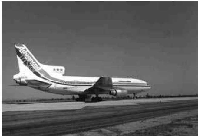
Lockheed L-1011, showing its rear engine installation. (Lockheed)
