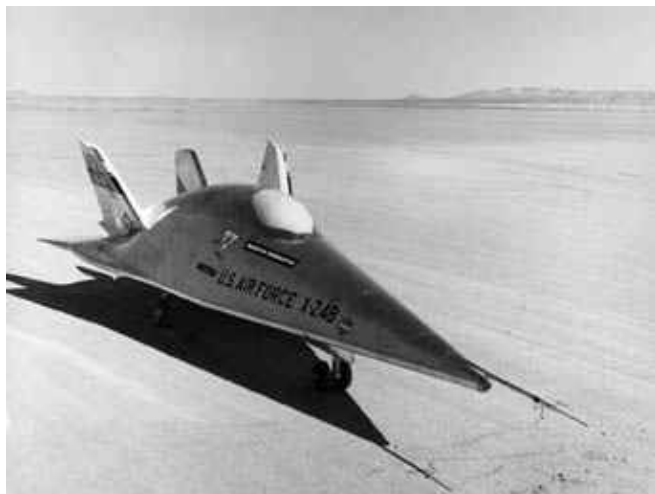
The X-24B, a lifting body capable of supersonic flight. (NASA)(E-25283)
