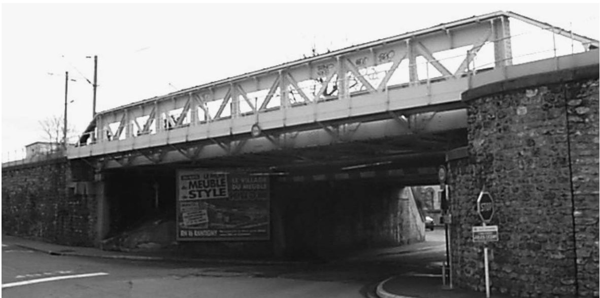
Fig. 1. The Gavignot bridge selected for the study.
