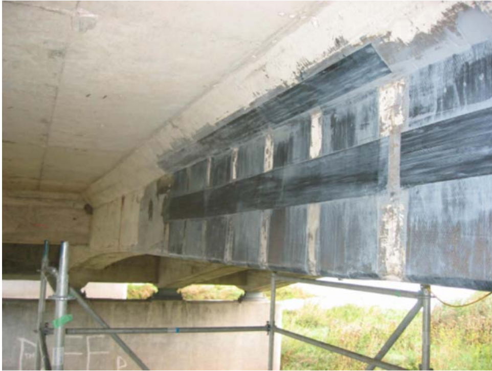
Figure 7. Photo of CFRP repair on the bridge girder
