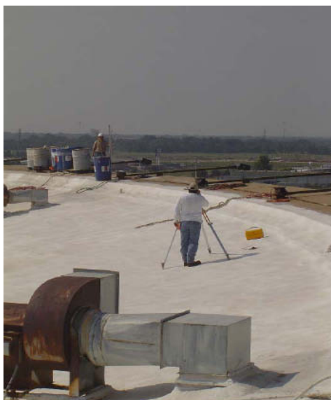
Figure 3. Surveying to determine roof sag.
