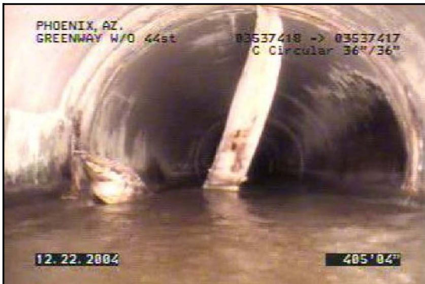
Figure 3. Detached weldstrip
