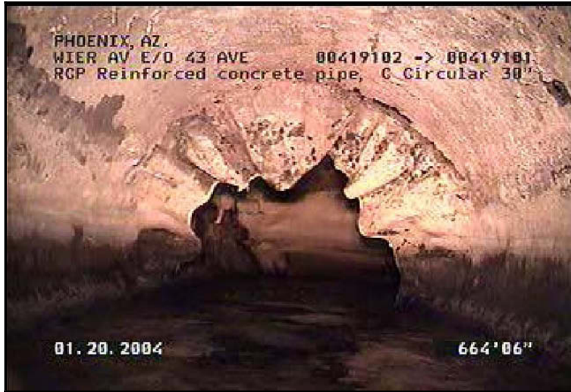
Figure 2. Detached liner
