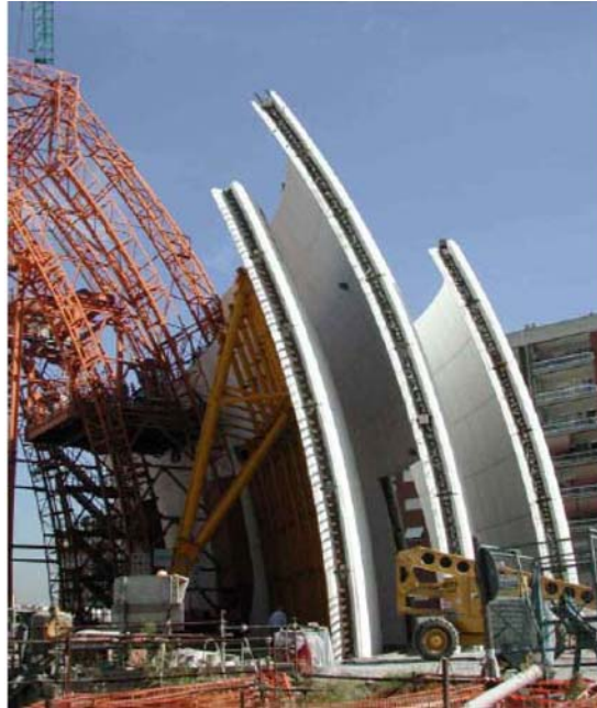
Fig. 1. The sail building phase of the “Dives in Misericordia” Church.
