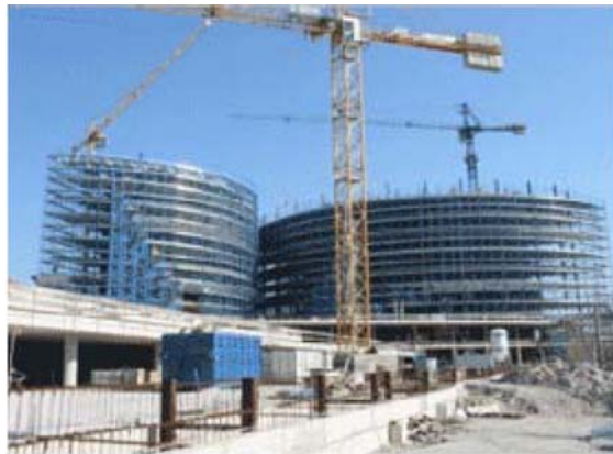
Fig. 2. WTC in San Marino construction site.
