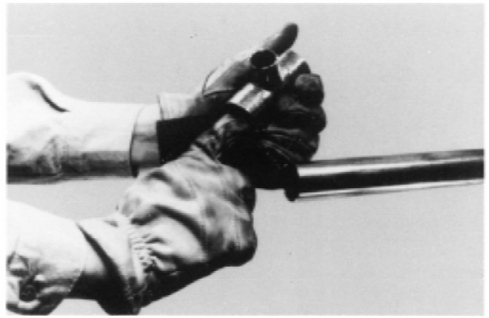
FIG. 8 Cleaning: Abrasive Pad
