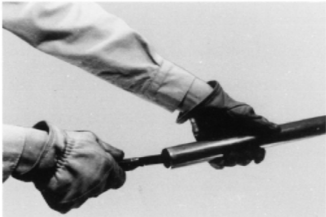
FIG. 4 Reaming: Pocket Knife
