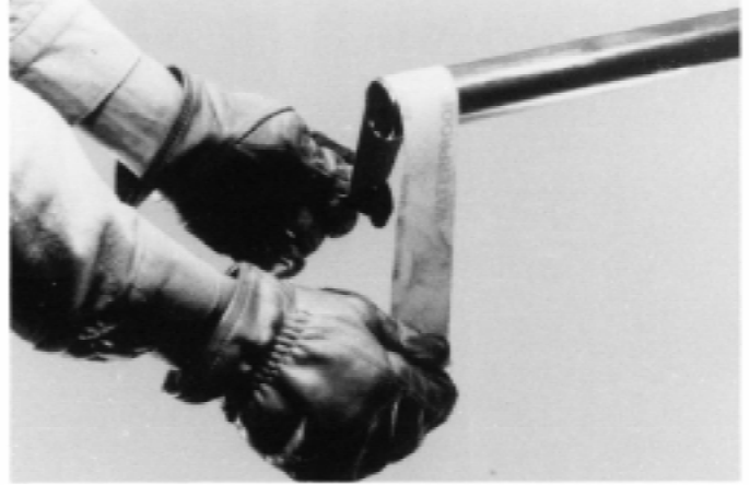
FIG. 6 Cleaning: Sand Cloth
