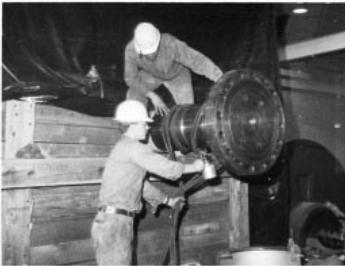
FIG. 8 Cable Magnetization
