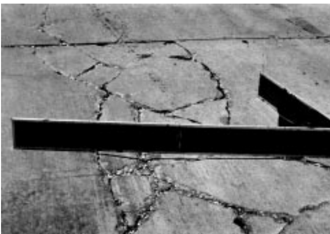
FIG. X2.37 High-Severity Punchout
