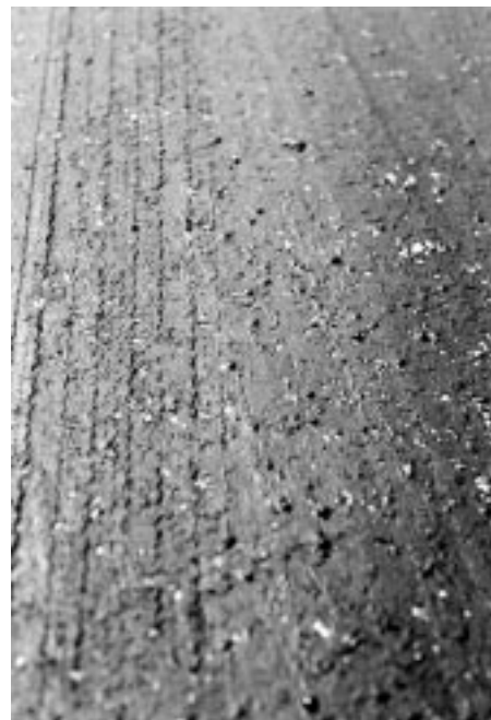
FIG. X1.6 High-Severity Bleeding
