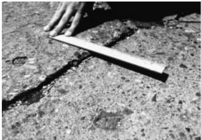
FIG. X2.14 Medium-Severity Faulting
