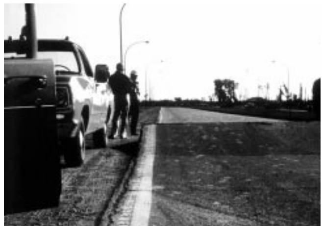
FIG. X2.3 High-Severity Blowup/Buckling
