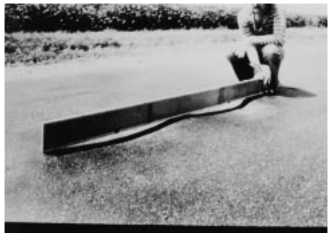
FIG. X1.15 High-Severity Corrugation
