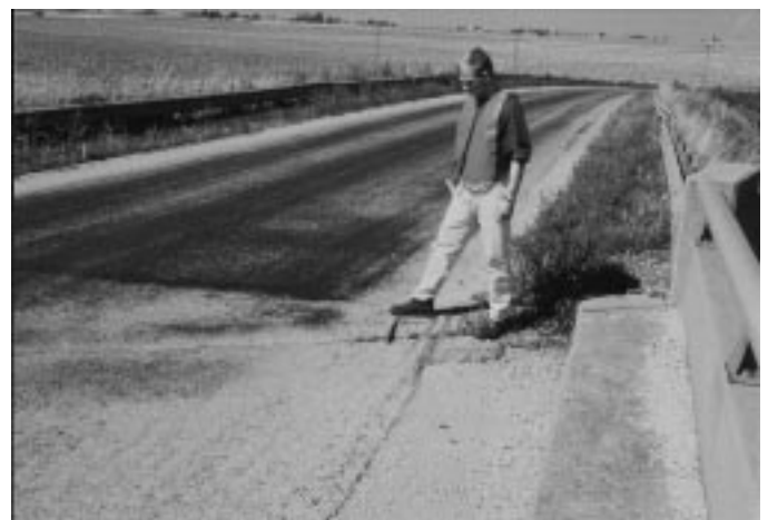
FIG. X1.44 Low-Severity Shoving
