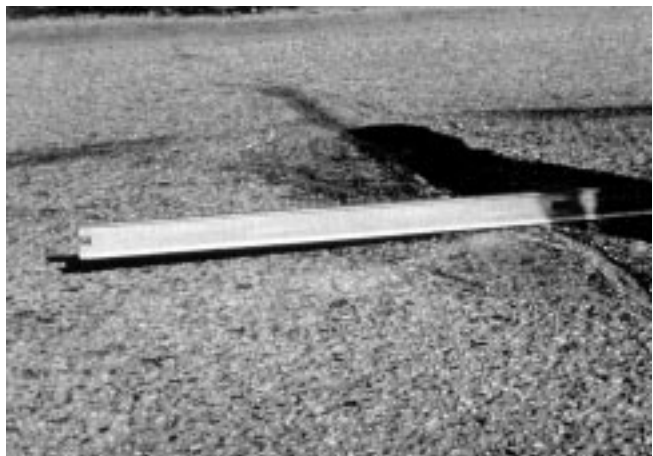
FIG. X1.10 Low-Severity Bumps and Sags
