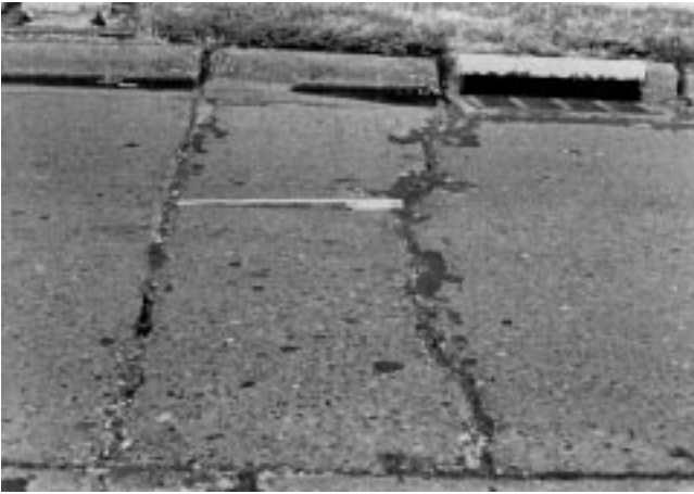
FIG. X2.35 Low-Severity Punchout
