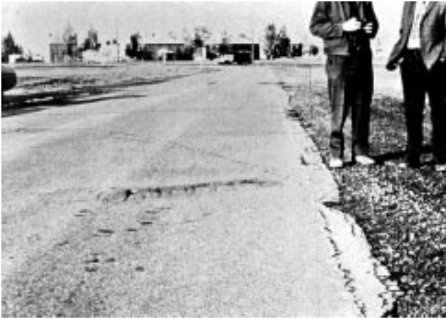
FIG. X1.11 Medium-Severity Bumps and Sags
