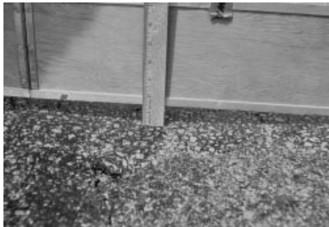
FIG. X1.43 High-Severity Rutting
