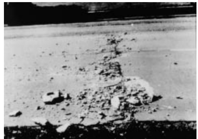
FIG. X2.2 Medium Severity Blowup/Buckling
