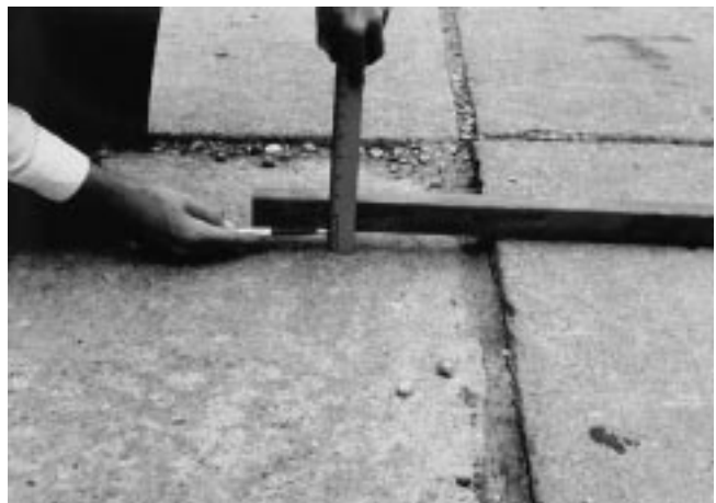
FIG. X2.15 High-Severity Faulting
