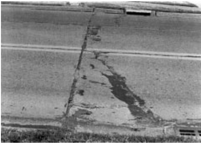
FIG. X2.36 Medium-Severity Punchout
