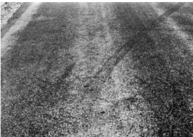
FIG. X1.4 Low-Severity Bleeding
