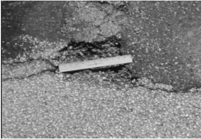
FIG. X1.35 Low-Severity Pothole
