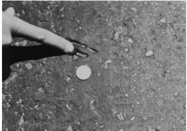
FIG. X1.5 Medium-Severity Bleeding
