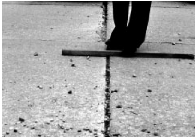
FIG. X2.13 Low-Severity Faulting
