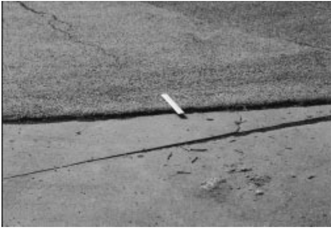
FIG. X1.45 Medium-Severity Shoving
