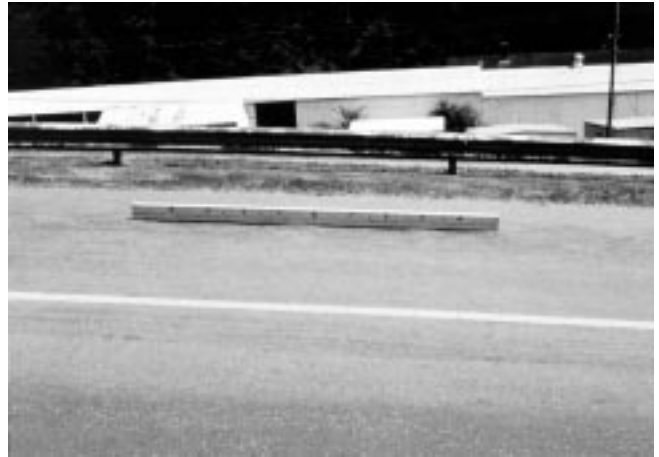
FIG. X1.14 Medium-Severity Corrugation
