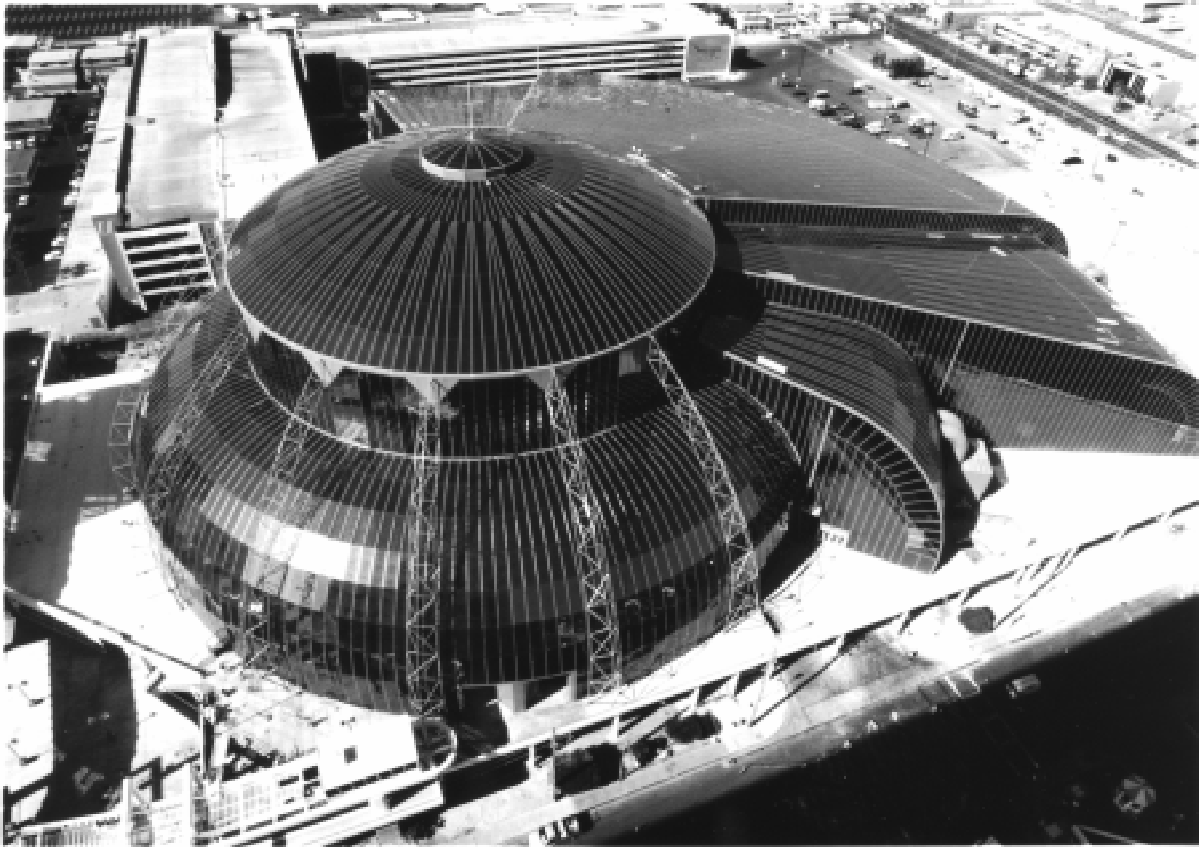
FIG. 5 Sloped SSG System
