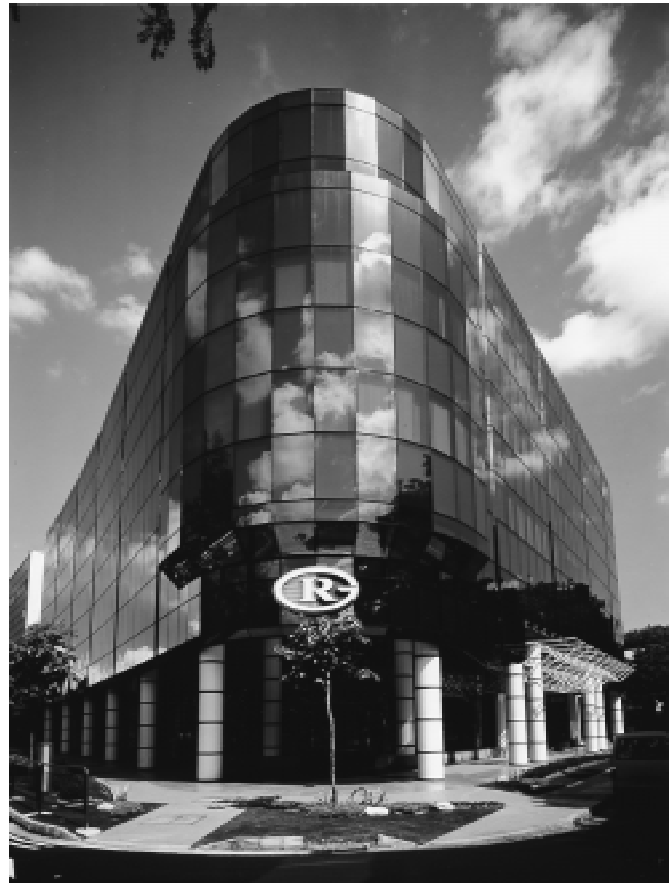
FIG. 3 Four-Side SSG System
