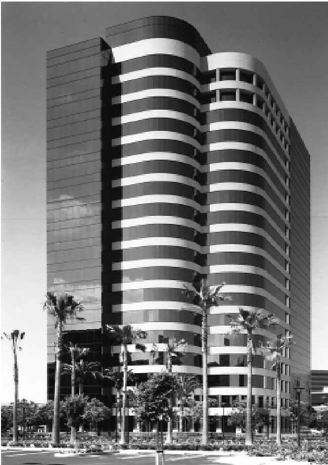
FIG. 2 Two-Side SSG System
