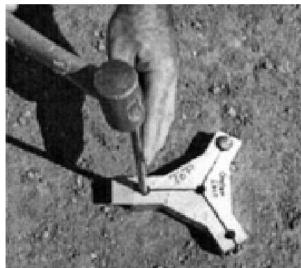
FIG. 5 Driving Spikes Through Template
