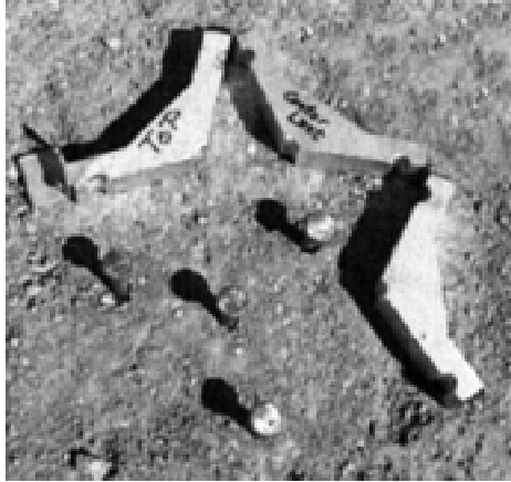
FIG. 6 Removal of Template After Driving Spikes
