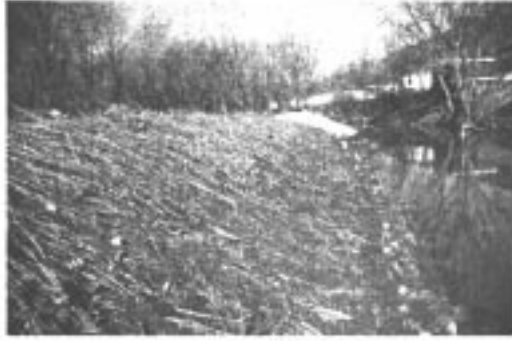
FIG. 1 Brushmattress after Light Backfill of Soil
