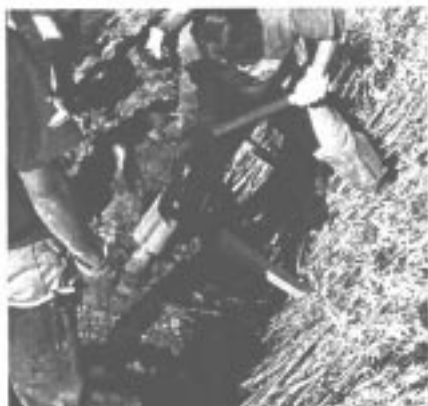
FIG. 5 Install Stakes Perpendicular to the Mattress
