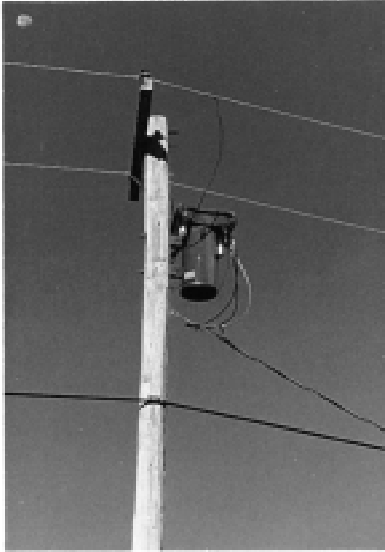
FIG. X2.3 Typical Pole-Mounted Transformer
