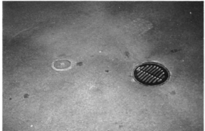
FIG. X2.5 Example of Floor Drain
