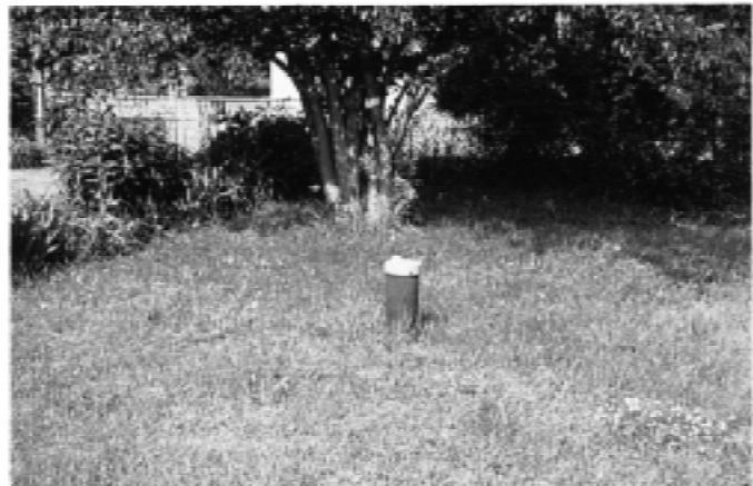
NOTE 1—Approximately 8-in. (203-mm) diameter. FIG. X2.10 Water Supply Well for Residential Property
