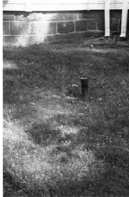
NOTE 1—Approximately 2½-in. (64-mm) diameter with screw cap. FIG. X2.9 Fill Pipe for Residential Underground Fuel Oil Storage Tank
