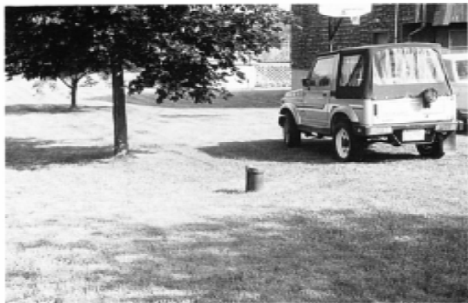
NOTE 1—Approximately 8-in. (203-mm) diameter FIG. X2.11 Water Supply Well for Residential Property
