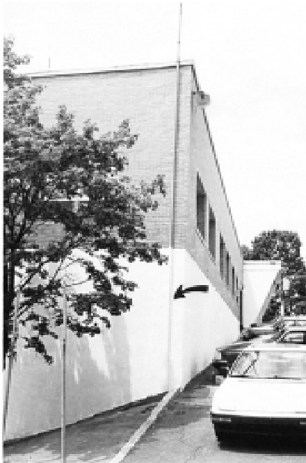
FIG. X2.8 Single Tall Vent Pipe (Arrow) for Underground Storage Tank on Side of Building
