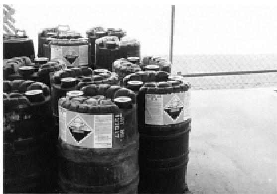
FIG. X2.2 Chemical Storage in 55-gal (208-L) Plastic Drums
