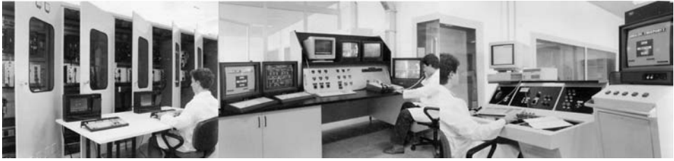
FIGURE 14.14 Control system: (a) level I of control system; (b) test facility control desk; (c) locomotive control desk.
